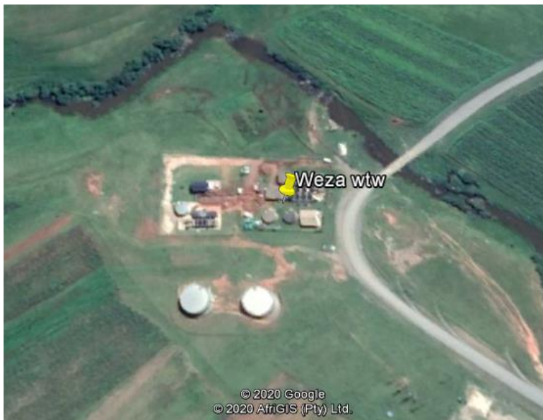
Existing Weza Dam
